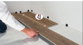
Figure 3: Use a full-length board for Plank 2 which will be installed in the second row. Align plank 2 at an angle, onto the long side of plank 1 making sure there are no gaps. Drop plank 2 to lock in place.
