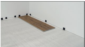
Figure 1: Planks should be staggered, with at least 8" (200 mm) or 25% of the length of the plank between end joint of adjacent planks. No plank less than 6" (150 mm) should be installed. Stagger planks to avoid installing in a brick like pattern on alternating rows. It is very important that the first two rows are installed properly. Installation will alternate back and forth between rows one and two, for the first two rows only. The first row of planks will be placed with the grooved edge facing outward into the room.
