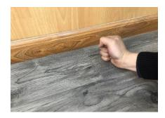
D. Using the drop lock system, drop the short side of the last long plank into the short side of the first laid plank. Slightly tap on the top of the joint of the short side with your fist to secure.
