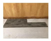
B. The first row must be installed straight. Begin installation back and forth between rows one and two for the first two rows only. Start small plank positioned close to the wall, angle a long plank into the long side of the short plank, and drop long plank tongue into lock. Make sure there are no gaps.
