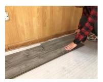
C. Take another long plank, repeat the previous step, insert the long side of plank into long side of previous plank. Then slide plank to your left until the short side is in contact with the short side of the first laid plank.
